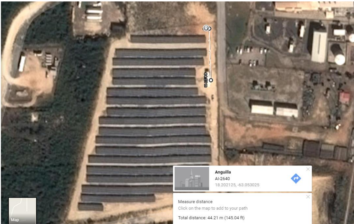
Image showing the approximate plan location of the battery system relative to the existing Ingeteam container
